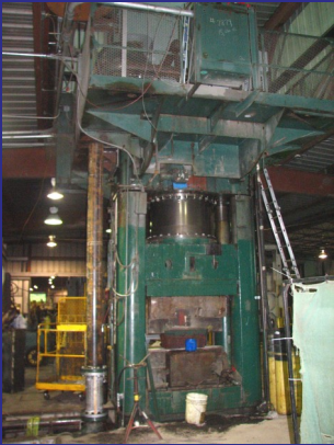
1500 TON PRESS WITH NEW PIPING
