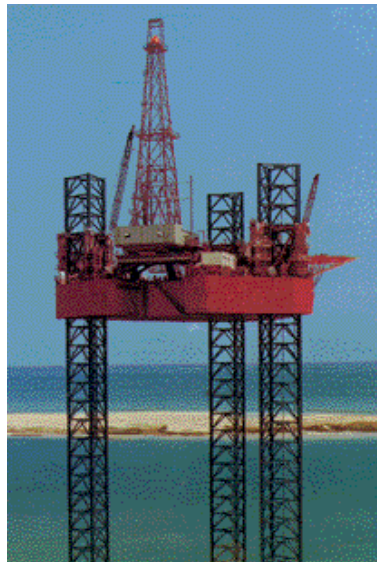
An offshore drilling rig with hydraulic jack up system
